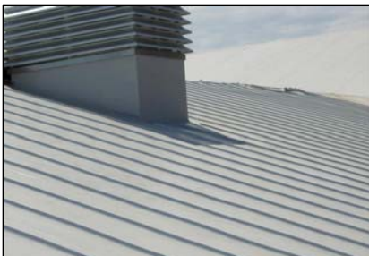
Vinyl Rib roofing system installed.
